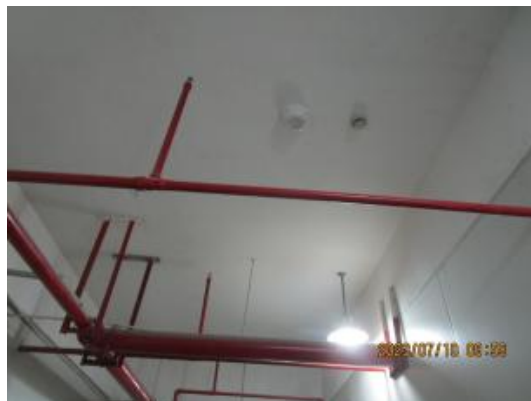
Sprinkler and smoke detector system.JPG
