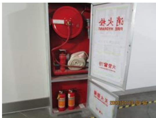
Fire hydrant and fire extinguishers.JPG
