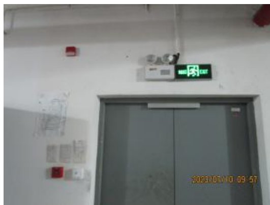
Exit sign, fire alarm and emergency light.JPG
